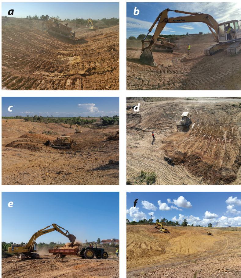
Figure 7. Geomorphic regrading actions: a), b), c) and d) Bulldozer and excavator constructing new rehabilitation topography; e) back-up tractors used for earth moving; f) view of the intervention area during late-stage of topographic regrading.
