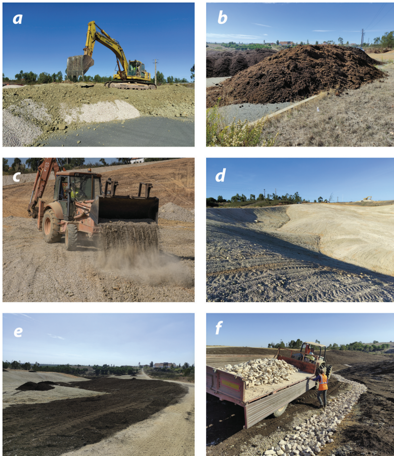
Figure 10. Execution of soil cover and AMD remediation actions: a) and b) materials used in the construction of the soil cover, limestone gravel and clays (a), and animal manure and topsoil (b); c) extension of the materials over the rehabilitation area with a backhoe; d) view of the intervention area after the extension of the soil horizon B; e) view of the first stages of the extension of the soil horizon A; f) lining of limestone blocks over the GeoFluv designed channels.
